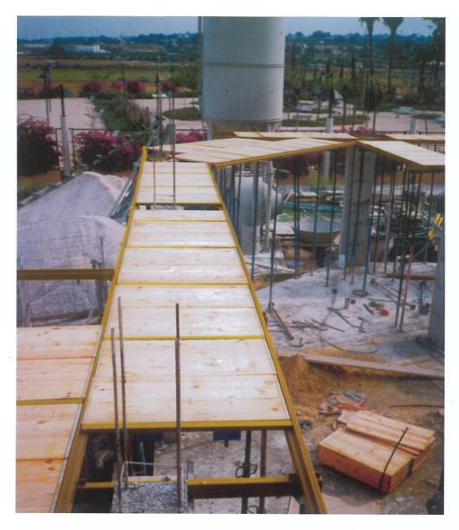
This horizontal shuttering system allows constructing ground beam structures easily and quickly.
