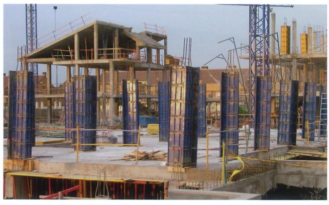
This kind of light formwork is perfect for column construction, with square or rectangle shape that requires manual handle (30x50 weight plate is 46 kg). Its special design makes possible the assembly with a small amount of accessories reducing the operators number to perform the placement to only two workers.
