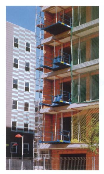
Maquiobras metallic platform eases the construction materials unloading at each floor of the building. It is recommended as a crane complement.
